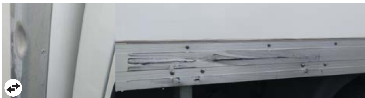
Underbody side profiles: Deformations within economic repair
