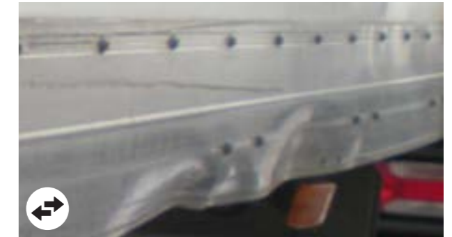
Underbody side profiles: Deformations beyond economic repair, perforations, removal of a section of the profile
