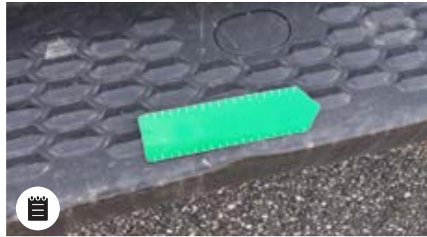
Rear Step Slight deformation
